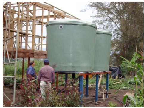
Des built the two new tank stands
